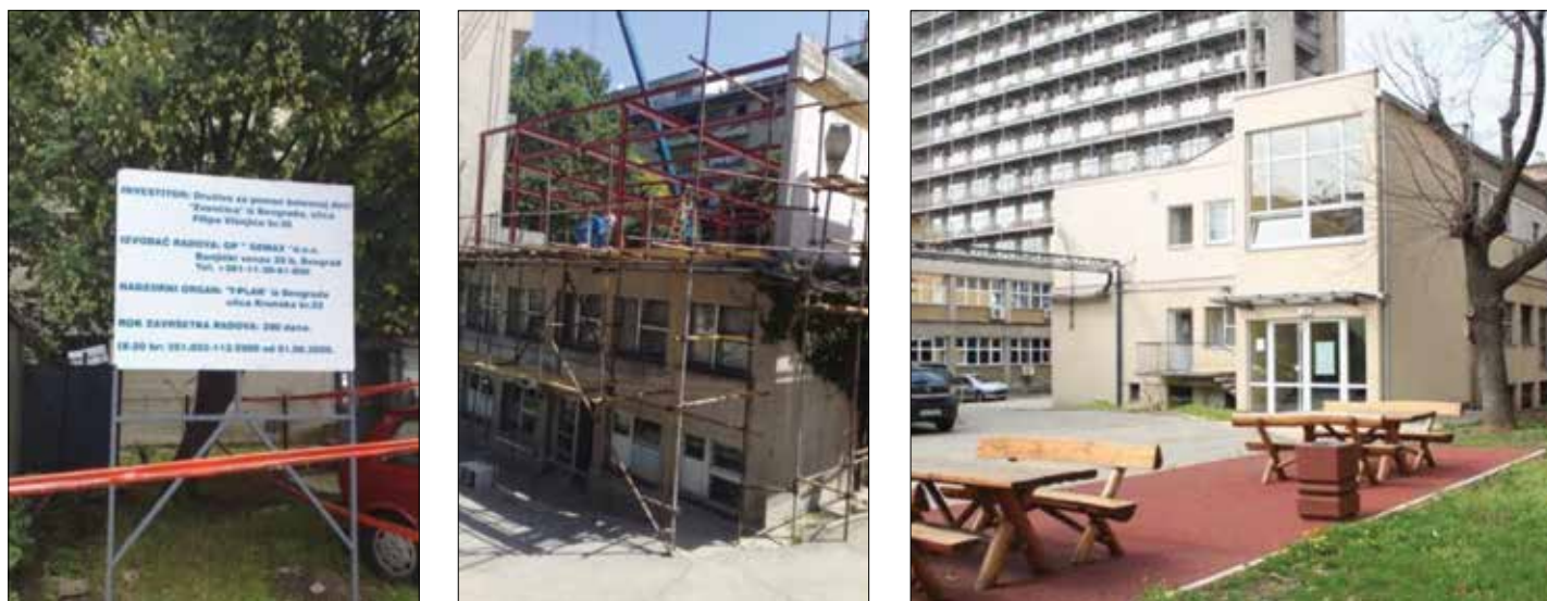
Figure 13. Construction of the Zvončica Parents' House
